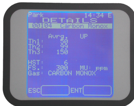
Figure 42) Detector details screen in "Engineer" level
